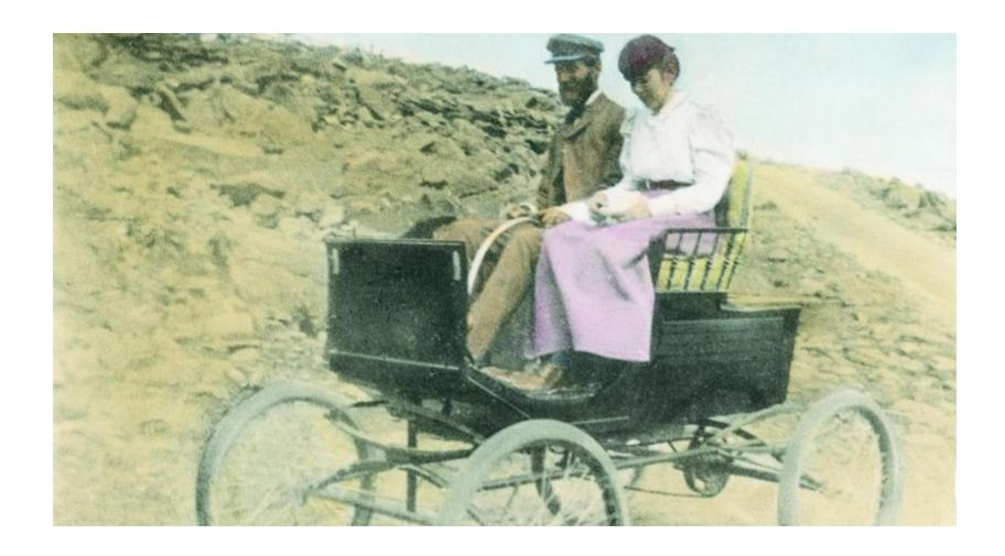
Vehicle is simply a light carriage, having a motor inside. Note "tiller steering" & rubber tire "bicycle wheels"
