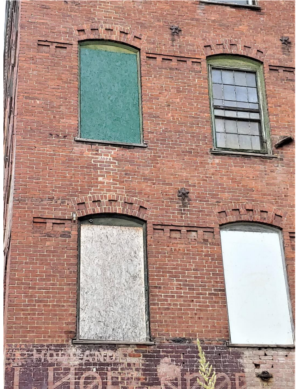
Lambert Hollander Building, first & second floor back windows, (1888)
