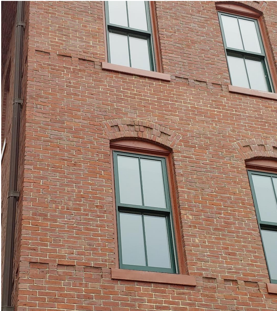
Convent second & third floor windows
